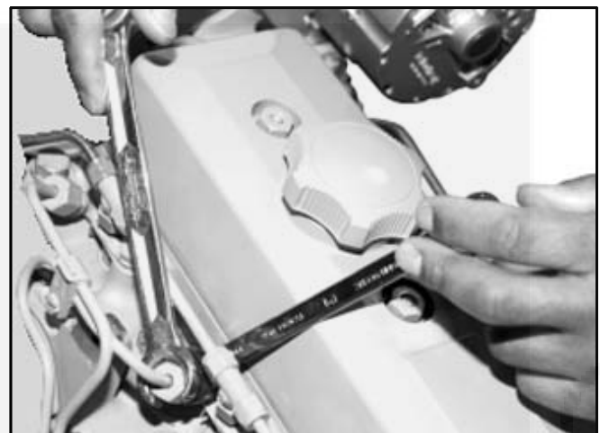
FIGURE 4-6. BLEEDING INJECTOR LINES
